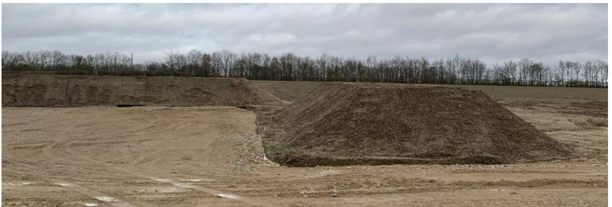
Photo 16: Topsoil Storage Example (Elsham – Lincoln Pipeline)
