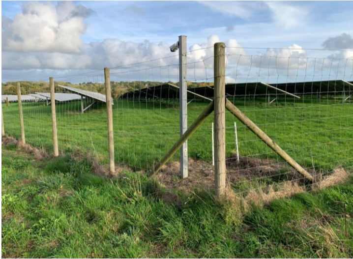
Photos 23 and 24: Typical CCTV Poles and Fencing
