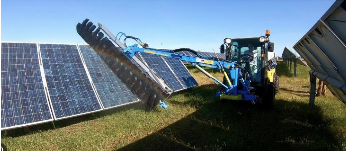
Photo 28: Cleaning of Solar Arrays
