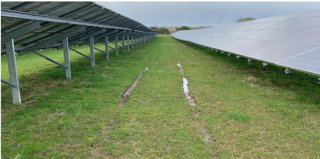
Photo 29: Ruts Caused by Vehicles
