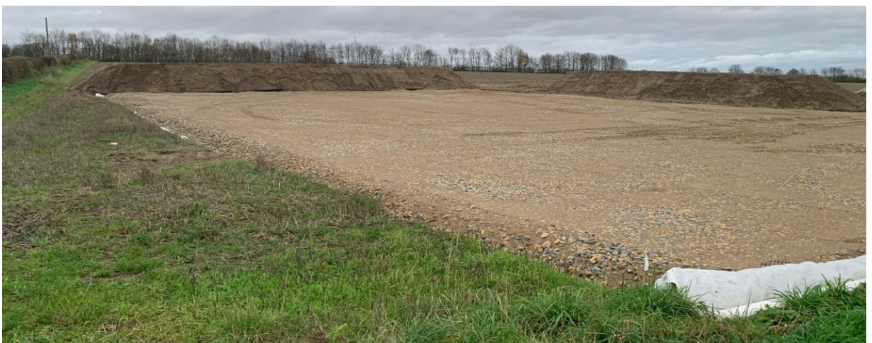
Photo 14: Newly laid Construction Compound (Elsham–Lincoln Pipeline)
