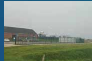
4 Indicative Satellite Substation***
