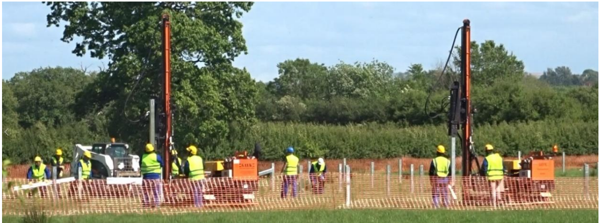
Photograph 15.7: Framework Posts being Installed
