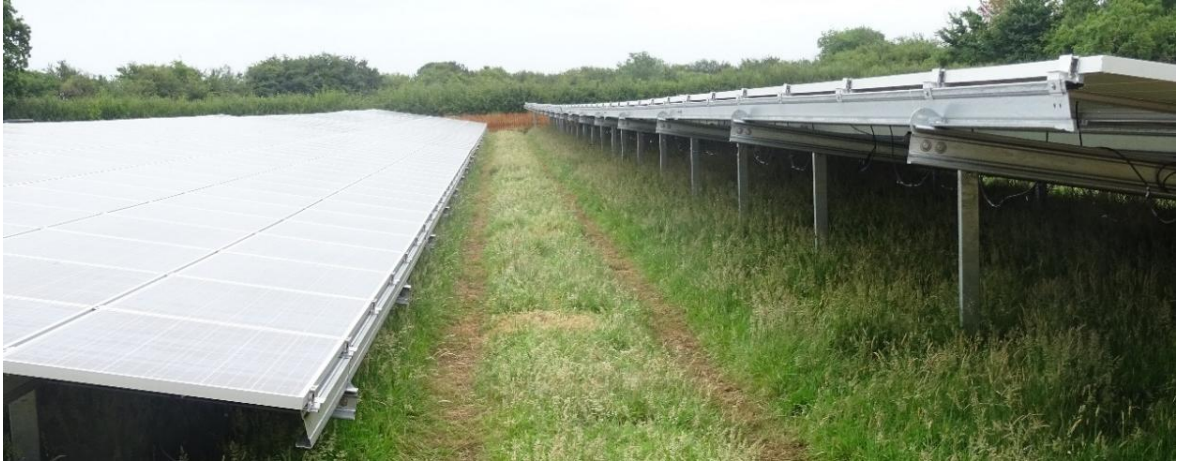
Photograph 15.10: After Solar PV Panels Bolted-on (Bentham Farm, Purton)
