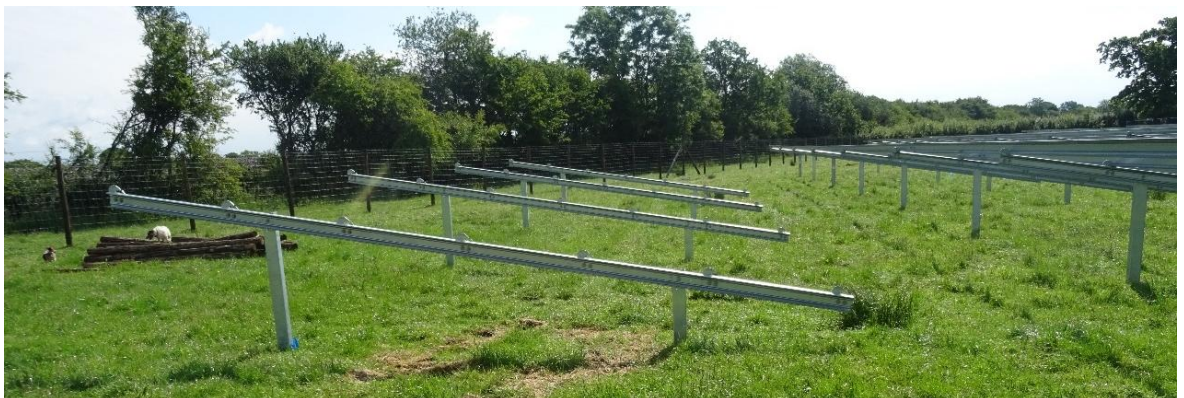
Photo 15.9: Framework Posts being Installed (taken at Tilm Farm, Retford, in January 2023)
